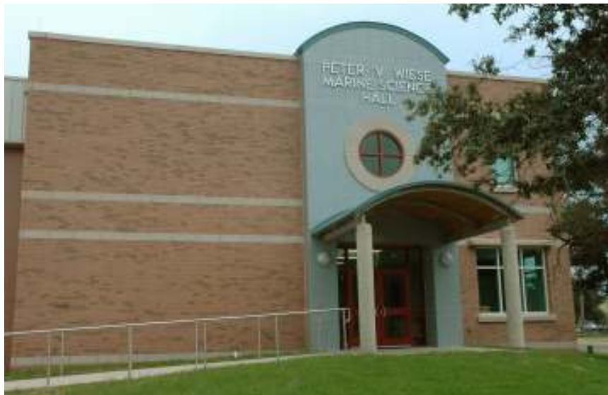
Peter V. Weise Marine Science Hall added 10,000 square feet in research and office space in 2006.
