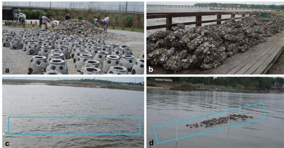
**Fig. 1** Photographs of project staging and deployment of (a, c) Reef Ball and (b, d) bagged oyster shell breakwaters
