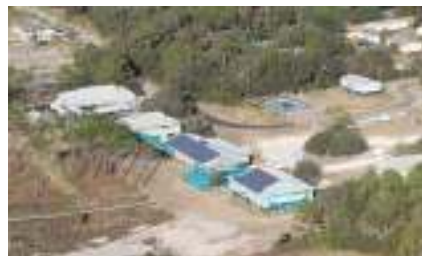
Solar panels, seen here on Horizon and Discovery Hall, have made the Sea Lab the largest public producer of solar power in the state of Alabama. Credit - John Dindo.
